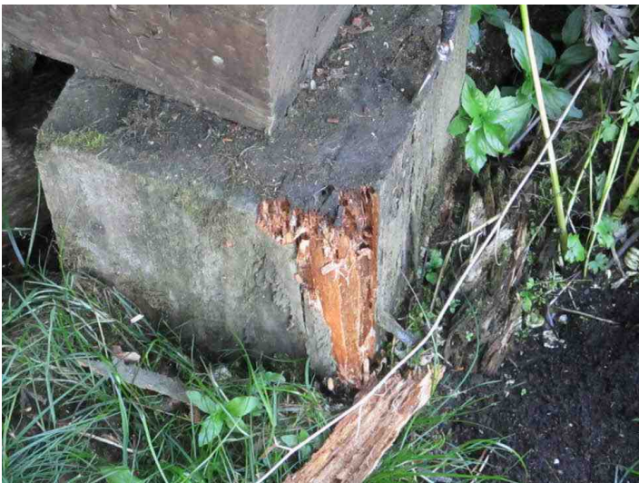
front porch foundation
