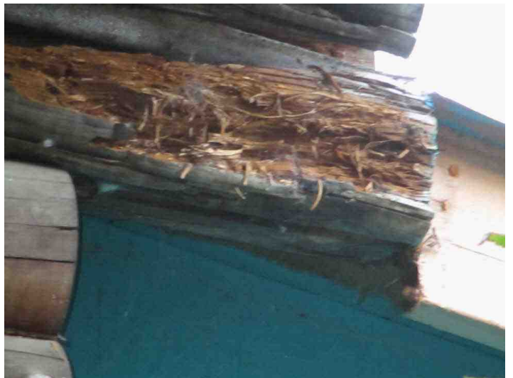
Logs to rear of house
